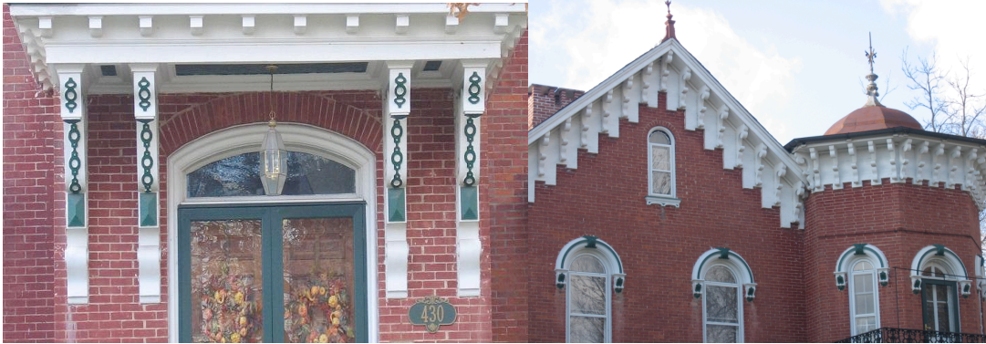
Details of brackets surrounding front entrance
